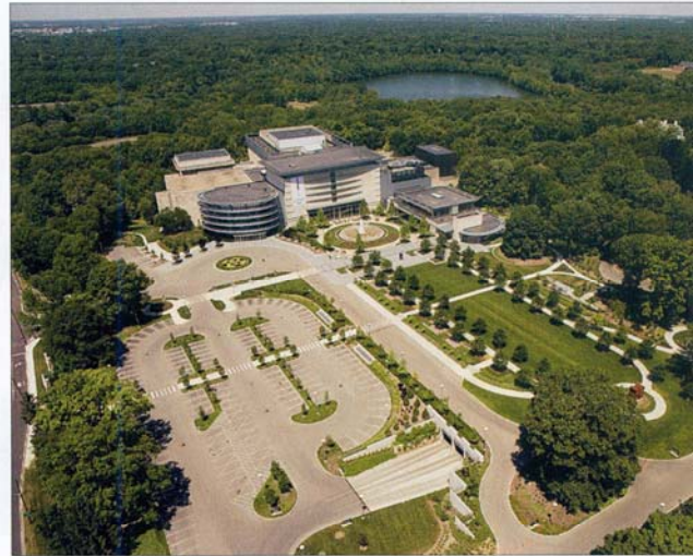
The Indianapolis Museum of Art features a parking garage with a roof garden that conserves energy and reduces storm-water runoff.
